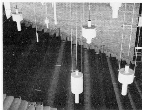
Figure 5.2: *Resonators and tubes from an installation in York [Parkin, 1970].*
